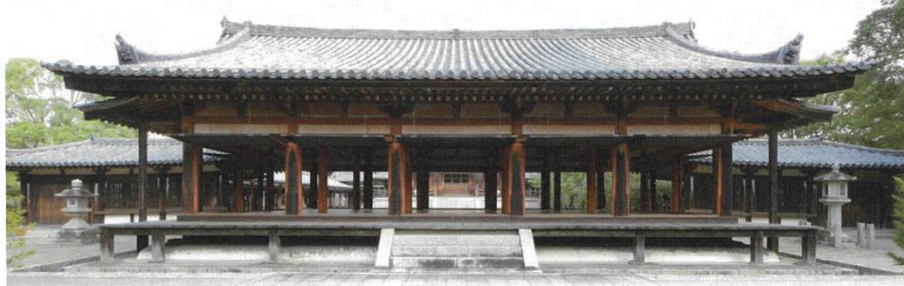
Facade before repair (from the south)
