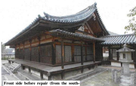
Front side before repair (from the south-east)
